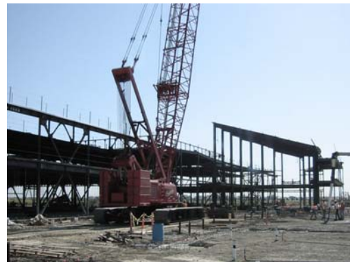
Construction of the new Inderkum High School
